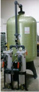
The ZeoMaxx and carbon filtration products are a family of mineral based medias offering the removal of a wide variety of water born contaminants. ZeoMaxx medias have high cation exchange capacities and can remove these and many other contaminants: Ammonia (NH<sub>4</sub>), heavy metals (Pb, Cu, Cd, Zn, Co, Cr, Mn and Fe; Pb, Cu as high as 97 %), toxins, low level radioactive elements (Cs, Co, Sr, Ag), flouride, oils, fuels, petrochemicals and others are adsorbed by ZeoMaxx.
